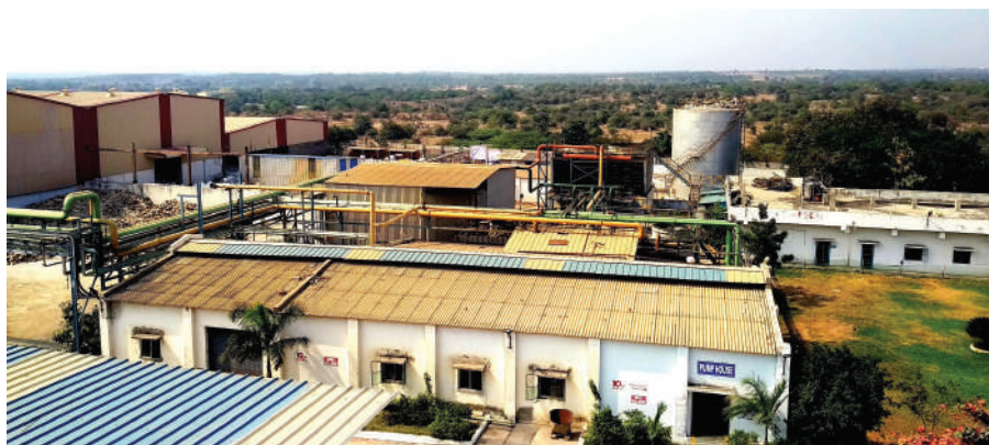
Future plant investments will see manufacturing capacity increased by 100%.
