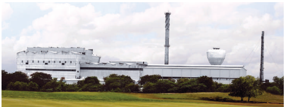
The Borosil Renewables factory at Bharuch, Gujarat.
