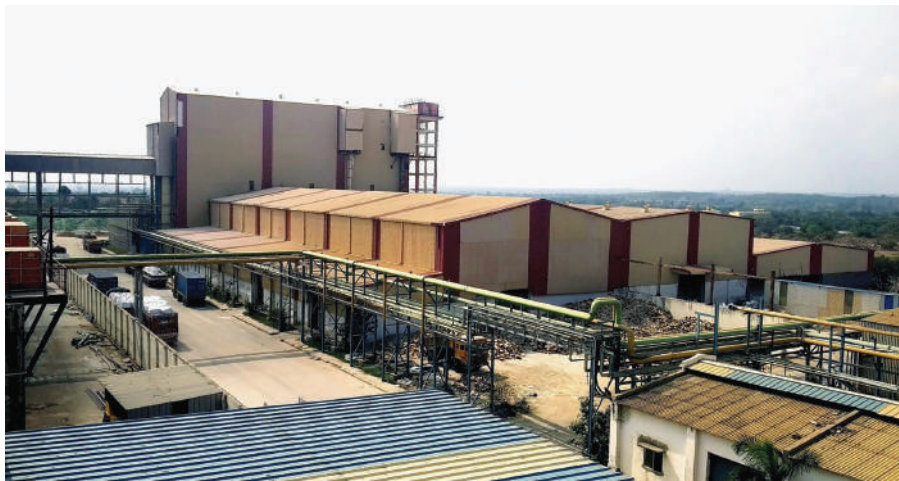
Both AGI glasspac plants have started using natural gas in their furnaces.
