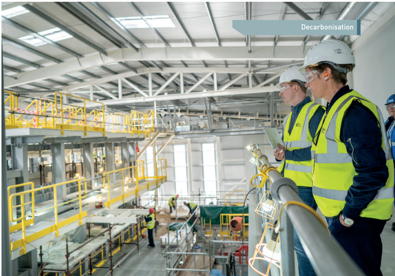
▲ Glass Future's pilot facility in St Helens, UK.
