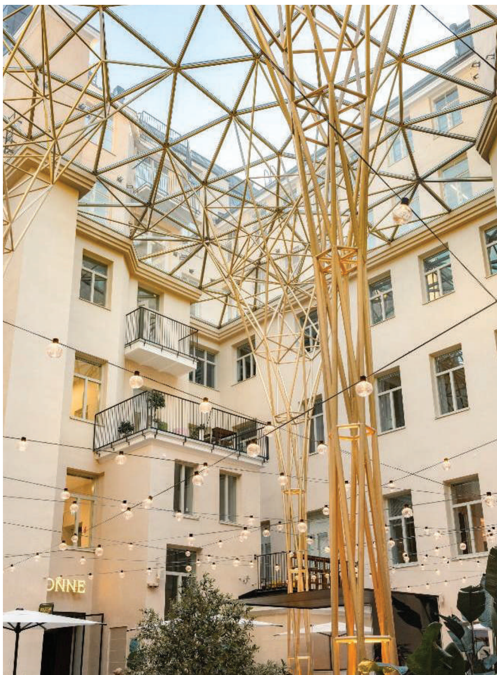
Four approx. 14m high steel columns branch out into a filigree structure that supports this glass roof. Photo: ©Jussi Hellsten
