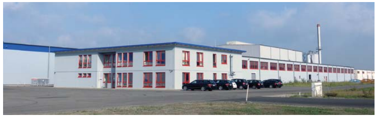
€50 million was spent on the greenfield glass container production complex at Gardelegen, Germany, sold to BA Vidro in 2016.
