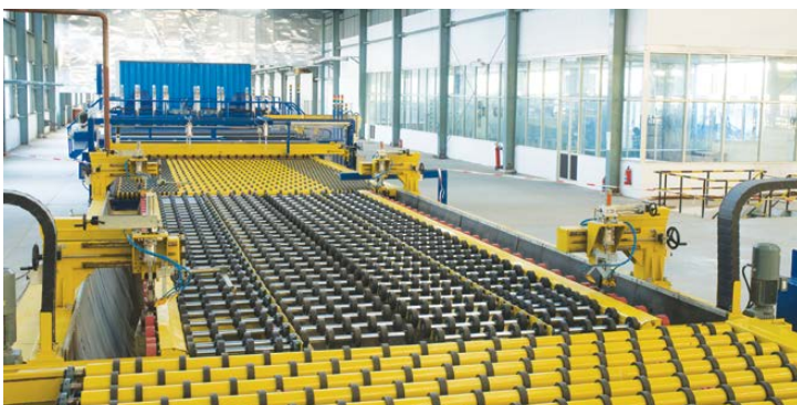
The Halol float glass project was completed within 21 months, making it the fastest execution within Indian glassmaking history.
