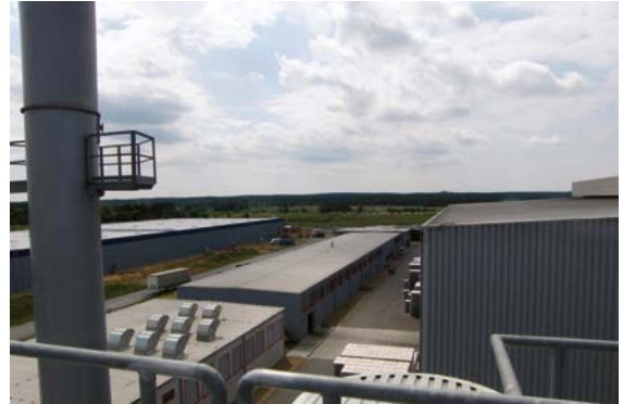
HNG's Gardelegen site concentrates on the production of white flint glass containers.
