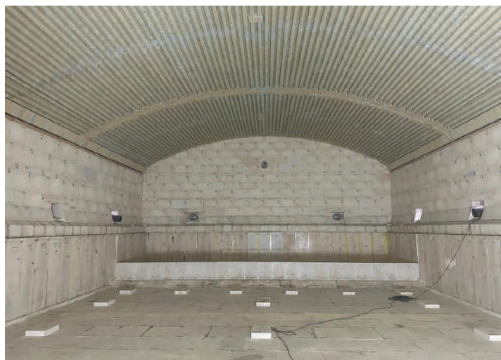
425tpd expansion project for AGI Greenpac, India.
