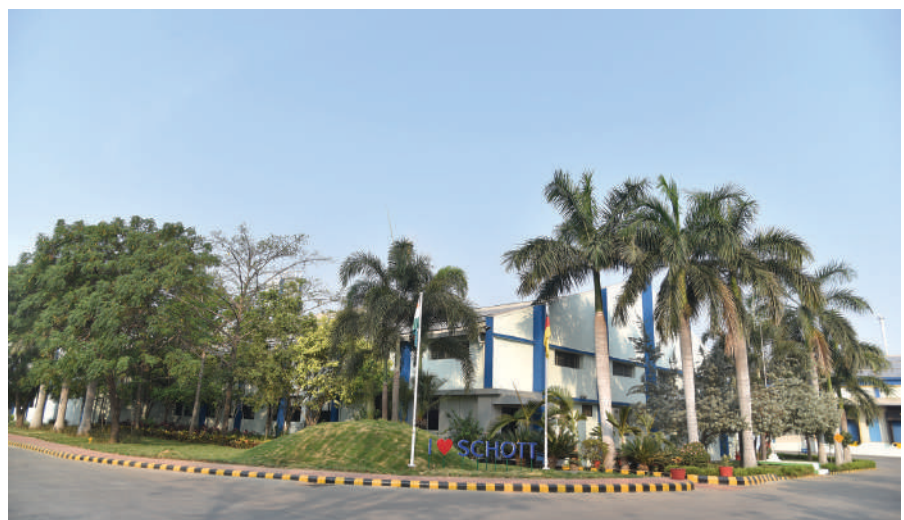
SCHOTT has invested €75 million to expand its pharma glass production in India.
