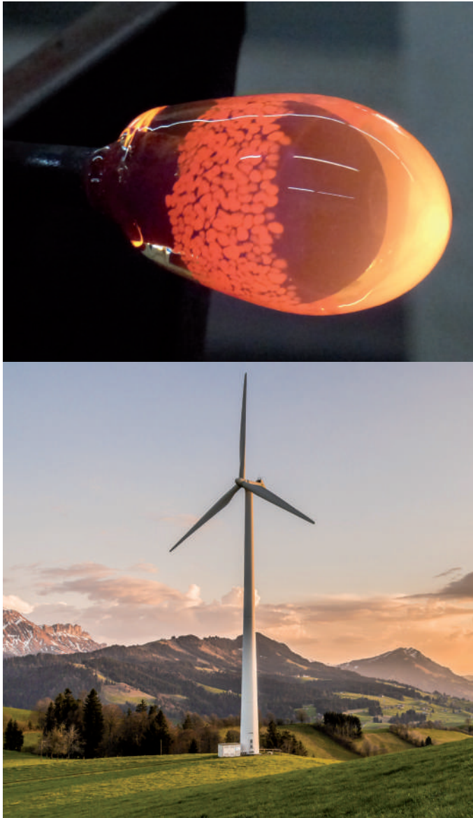
Figure 6. The blades of wind turbines are reinforced plastics using glass fibers with a high Young's modulus.
