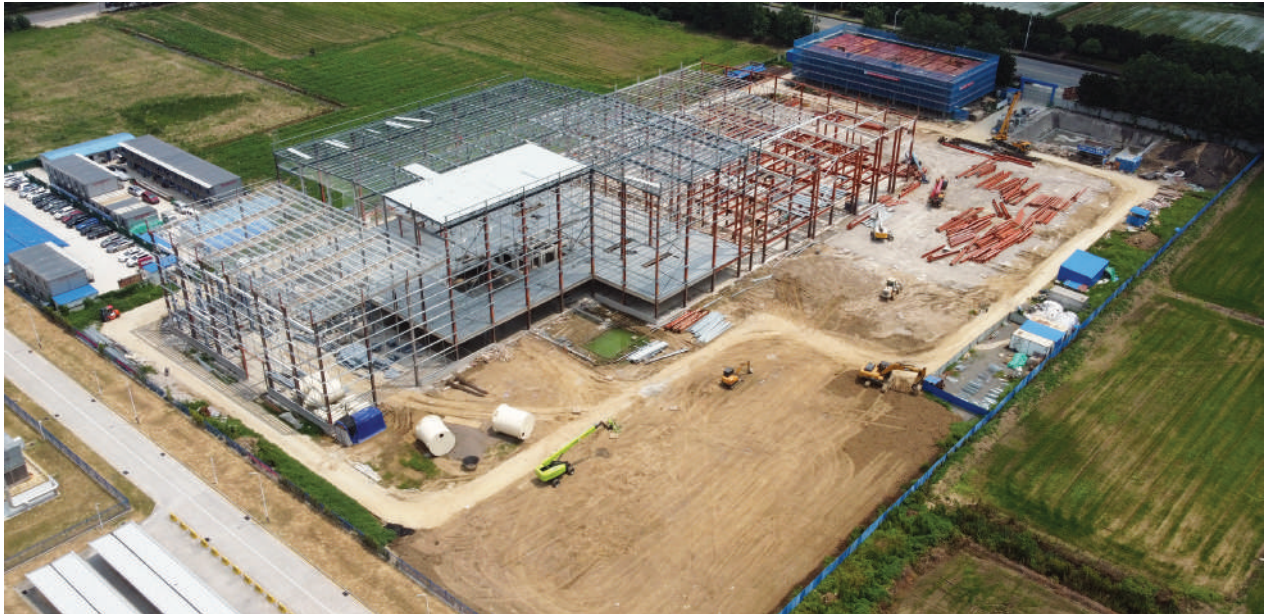
The greenfield construction site in China.
