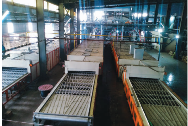
Annealing lehrs during installation at the Behror glass container plant.
