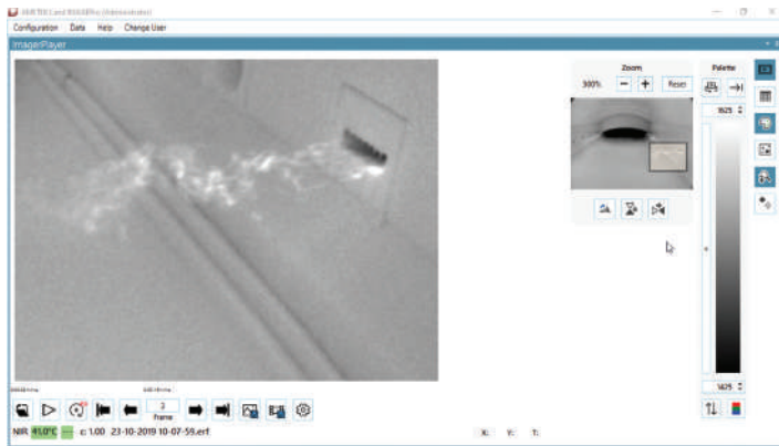
Continued operation will most likely see damage to the L4 block on the bottom downstream corner.
