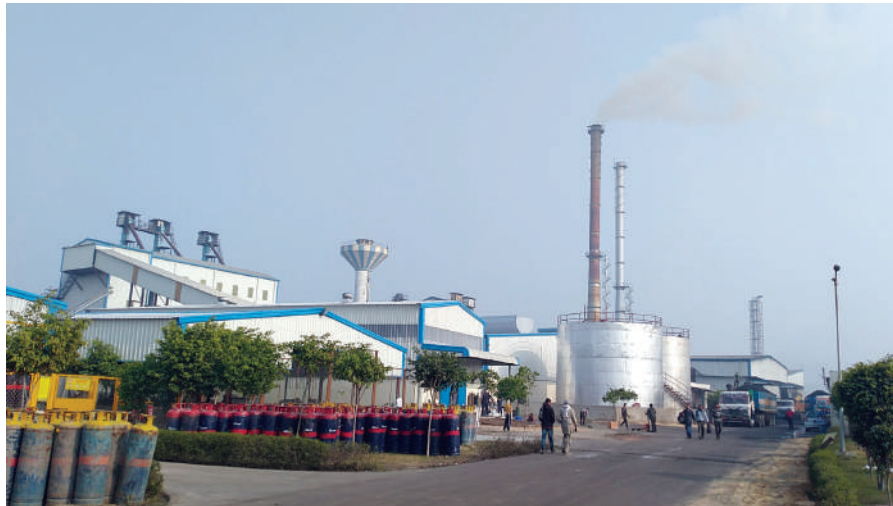
The Emerge Glass site in Rajasthan houses a recently completed glass container factory.
