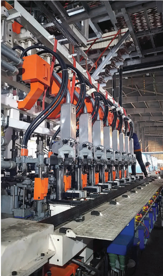
Four advanced IS machines have been acquired from Shandong Sanjin Glass Machinery Co Ltd.
