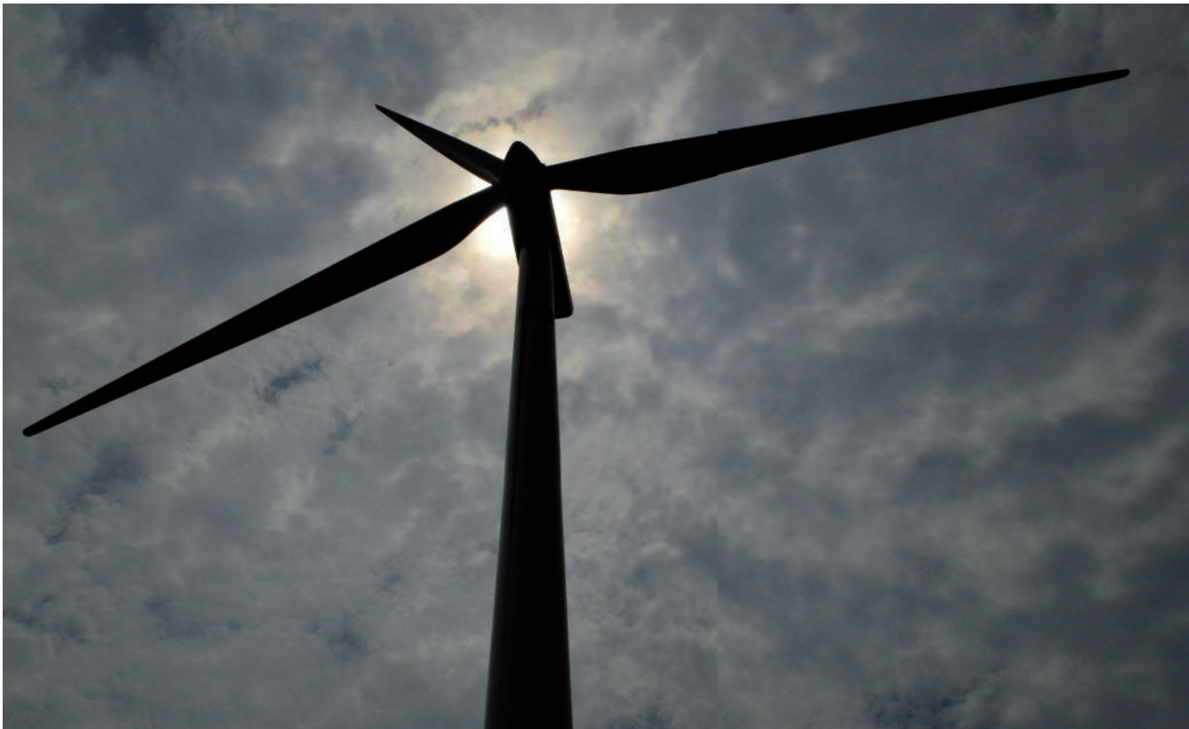
Figure 6. A stunning image of a wind turbine
