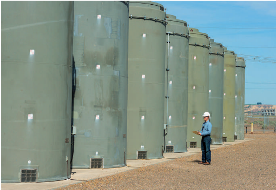
Figure 7. Used nuclear fuel is stored above ground in massive airtight steel or concrete-and-steel dry canisters, or in steel-lined water-filled concrete pools
