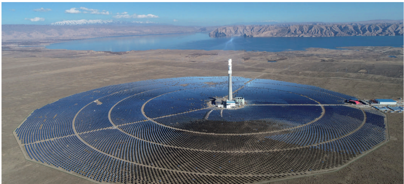
Figure 4. 50MW Solar Thermal Power Plant in Qinghai, China
