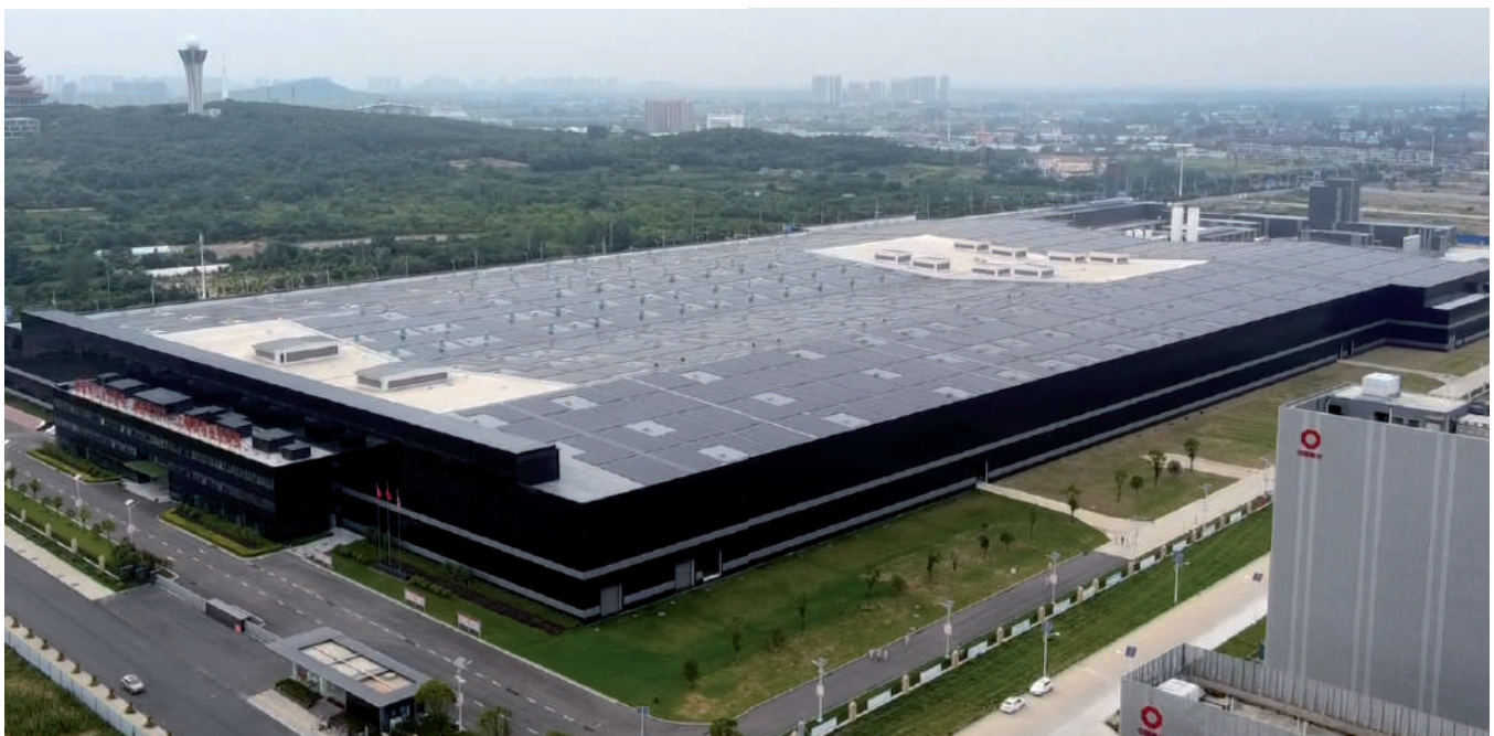
Figure 1: World's largest integrated thin-film solar cell building demonstration project in Anhui, China
