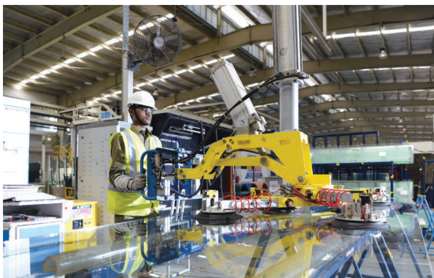
The ‘World Glass Complex’ near Chennai is the largest float glass plant in India.
