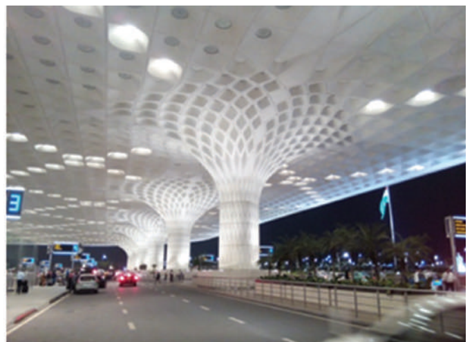
Panels in T2 international Airport, Mumbai
