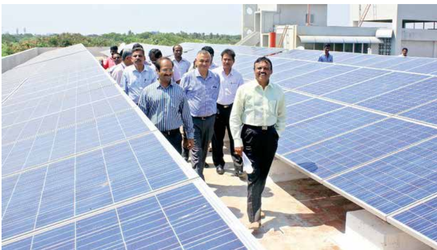
Fig. 7: 110 kWp Solar Plant installed at General Pool Office Building at Chennai
