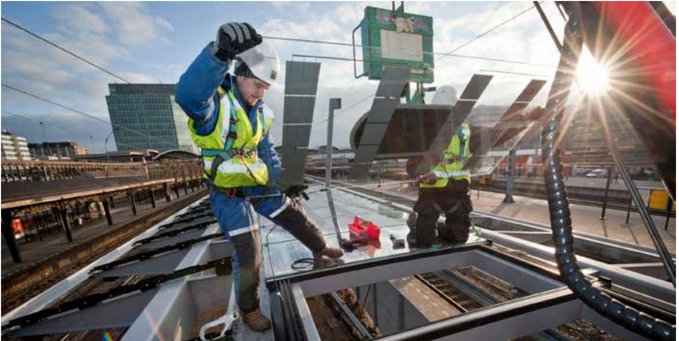
Dual benefit: In railway stations BIPV panels are seen ever more often. They serve as sun screens while supplying clocks and display panels with power at the same time. Photo: ertex solartechnik
