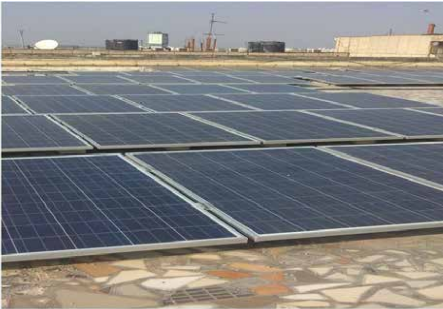
Fig. 5: 100 KWp Grid Interactive Roof Top Solar Power Plant at Sewa Bhawan, R.K.Puram, New Delhi
