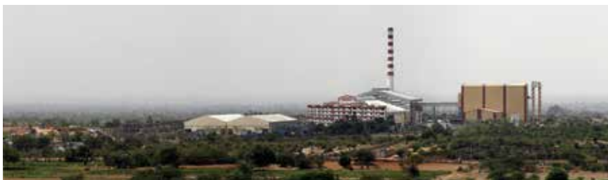
The AGI facility in Bhongir was commissioned in 2009 and a new furnace was constructed in 2013.
