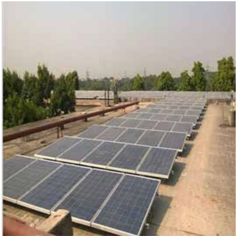
Fig. 3: 500 KWp Grid Interactive Roof Top Solar Power Plant at Pushpa Bhawan New Delhi
