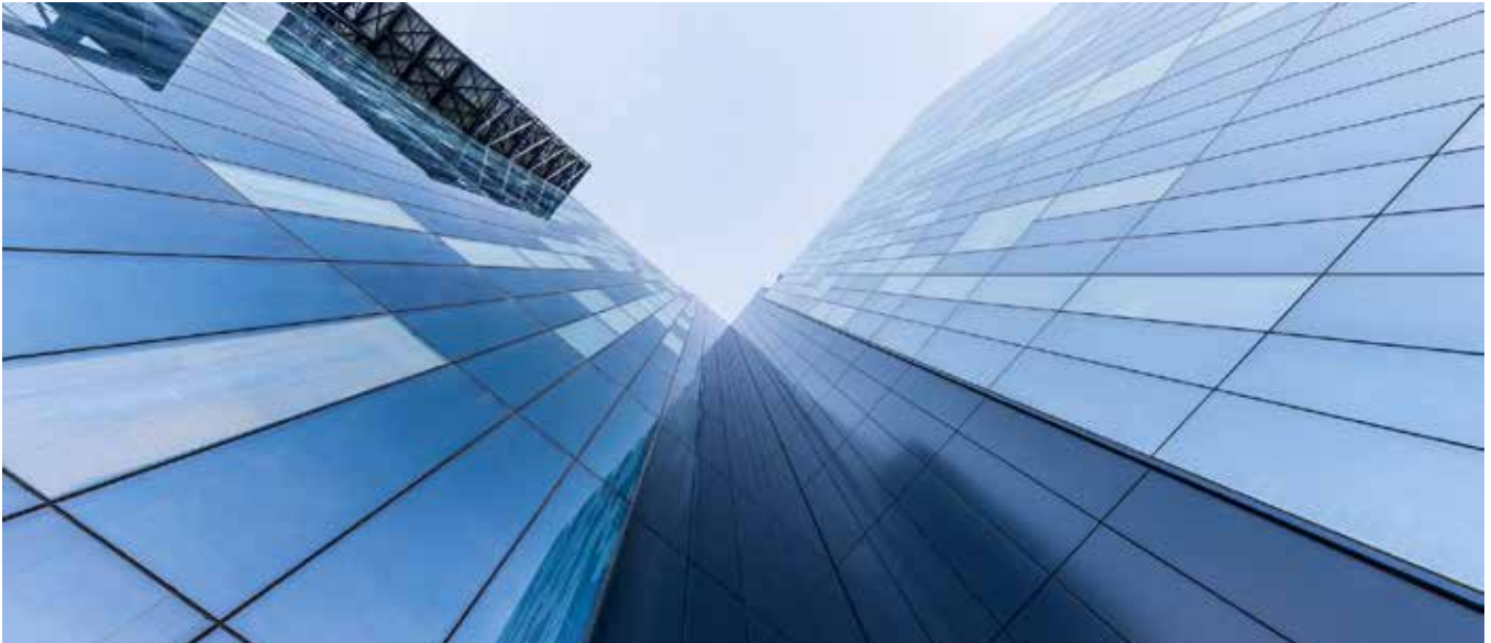
Major project: Transparent films can also be laminated between window panes. The result is tinted glass panes that provide shade and generate green electricity at the same time. Photo: AGC Glass Europe, Louvain-la-Neuve
