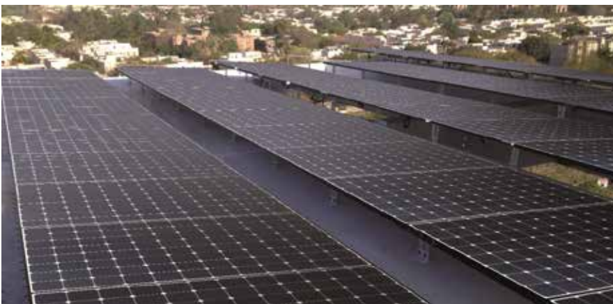
Fig. 6: Solar Rooftop Panels in Indira Paryavaran Bhawan, New Delhi installed during construction
