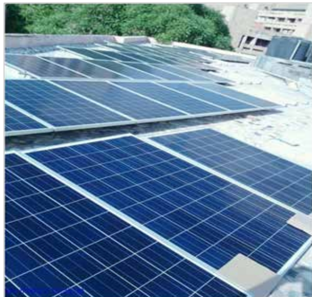
Fig. 4: 250 KWp Grid Interactive Roof Top Solar Power Plant at East Block R.K. Puram, New Delhi
