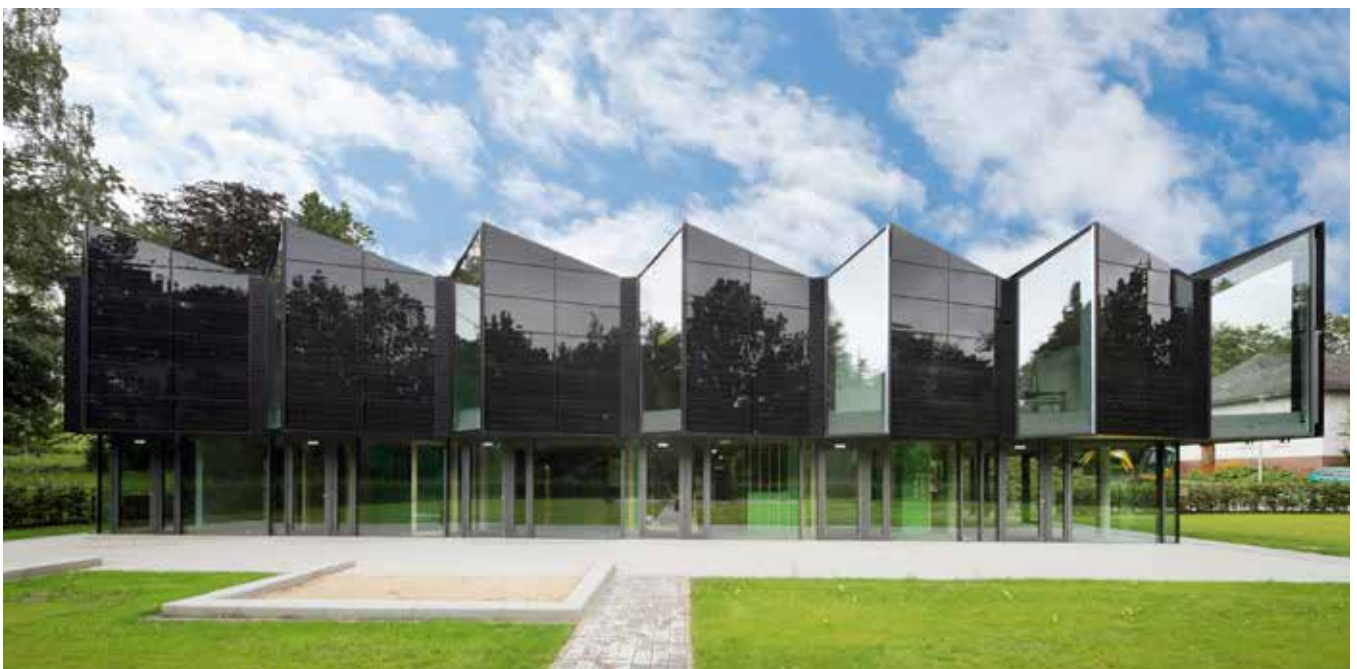
Showcase project: The main façade of “E+ Kita Marburg” consists of special solar modules in black laminated safety glass which perfectly blends in with the overall architectural look and feel. Photo: ertex solartechnik
