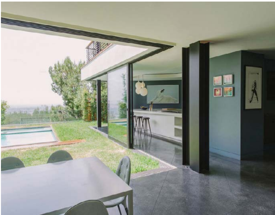
Frameless Glass Wall - Green Greenberg Green House, Los Angeles, USA – LEED Silver [1]
