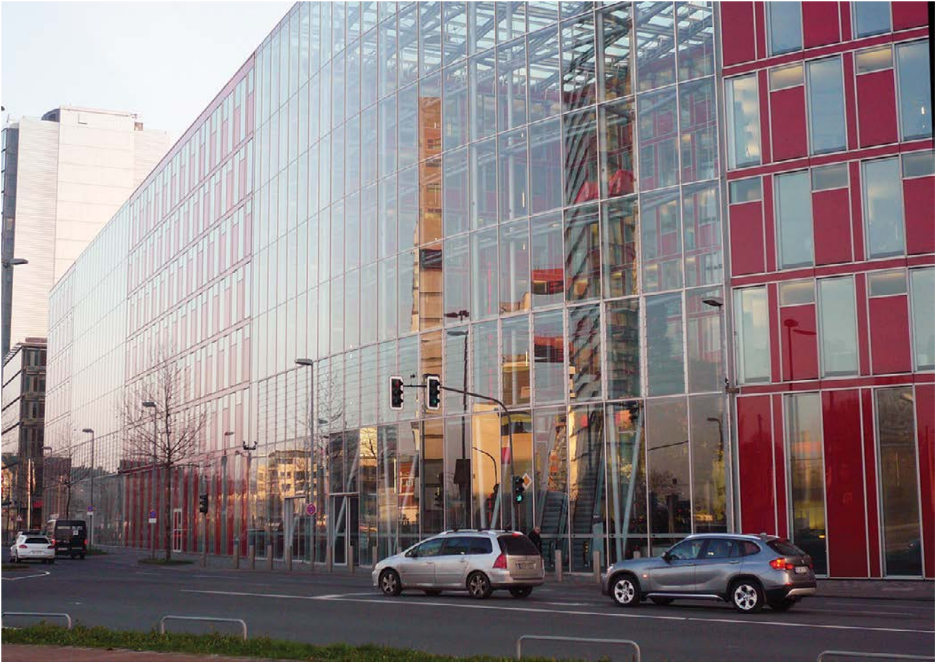
The Capricorn House in Düsseldorf was finished in 2006 and has been awarded the Innovation Prize for Architecture and Office, and the label “best architects 2008”. One design highlight of the building is the i-module facade. Integrated modules cool, ventilate and reclaim heat. In addition, lighting, sound absorption and room acoustic elements are integrated in the façade panels.
