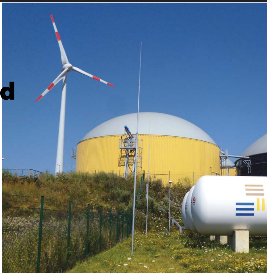
'Wind gas' plant produces hydrogen from excess wind power and mixes it with biogas to produce electricity. Hydrogen can also be stored and used to run cars
