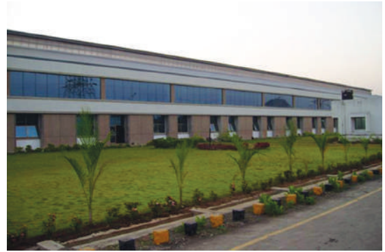
AIS refurbished its existing Taloja float glass facility in 2018.
