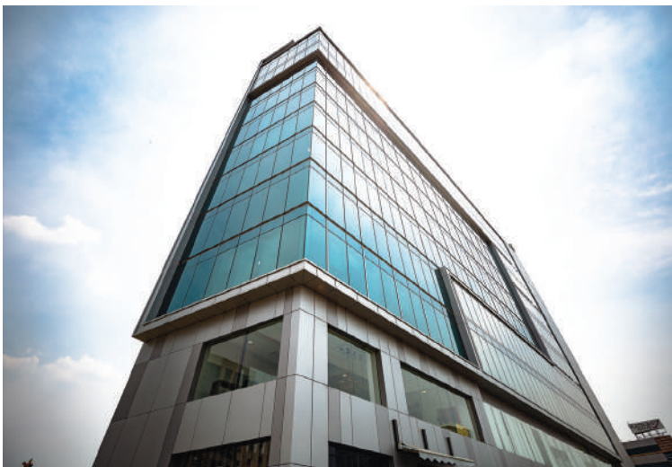
Aihant, The Verge in Chennai uses Saint-Gobain’s Planitherm Clear (Planitherm – Pristine White), KT440 (Nano – Tropical Green) and ST436 (Cool Lite Turquoise) glass materials.
