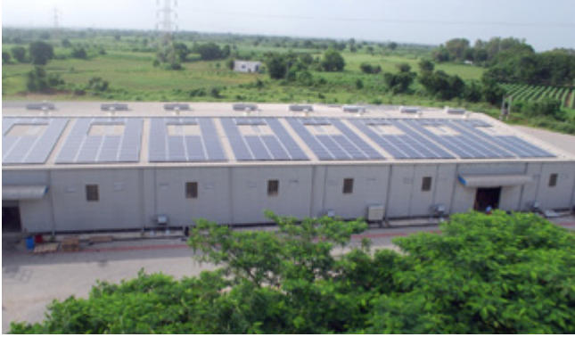
Fig.4:PV module arrays at Vyline Glass Works, India with Antimony and Antimony-free glass modules
