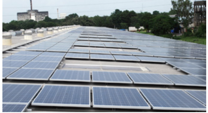
Fig.5: Installation of PV module arrays at Vyline Glass Works, India with Antimony and Antimony-free glass modules
