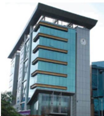
Fig. 12: RTI Building, Mumbai
