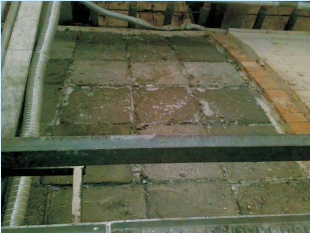
Fig. 1: Large area of a float furnace crown sealed with Lubisol Si-Seal kit
