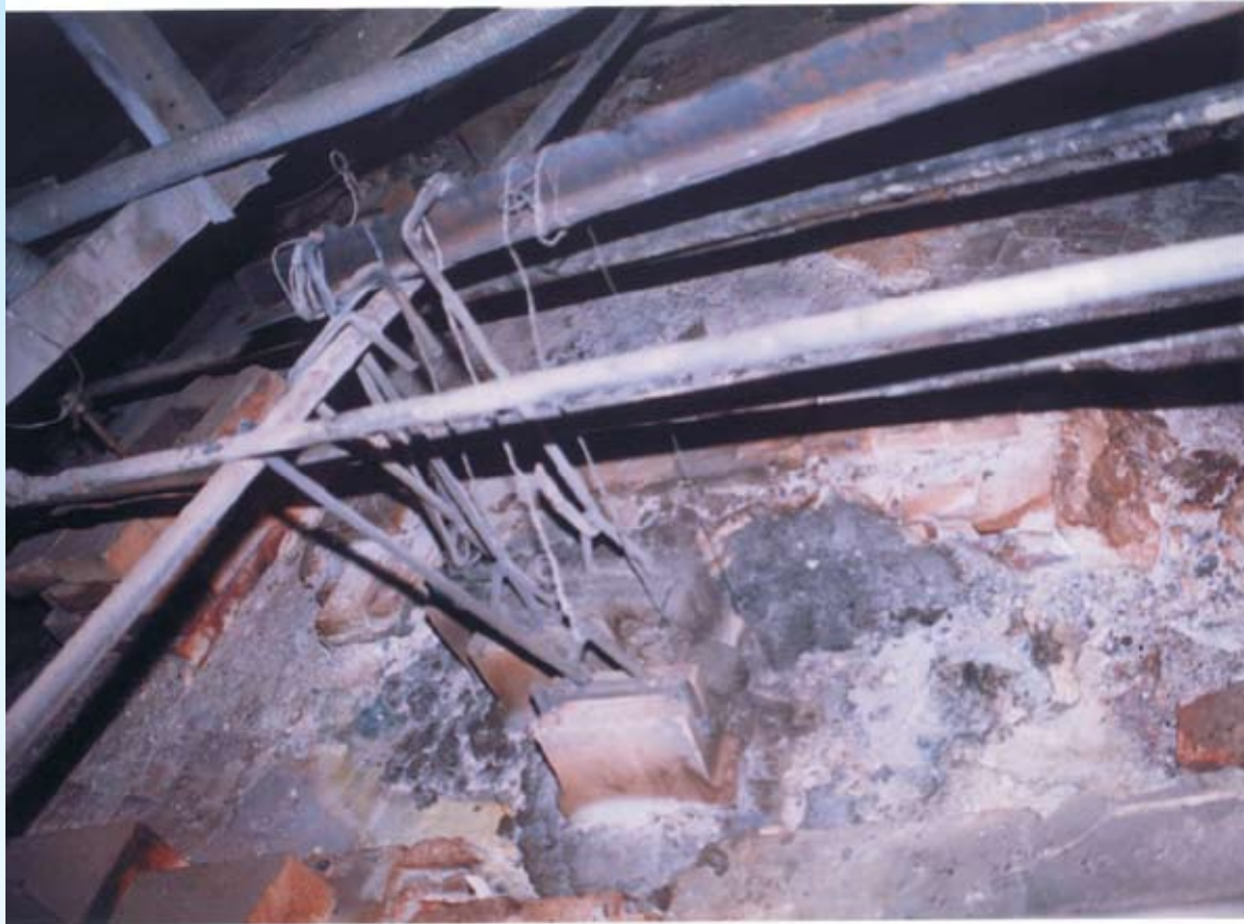
Fig. 2: Hot repair of a container glass furnace with suspended fused silica blocks and Si-Seal kit
