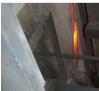
Transition brick port neck before ceramic welding.
