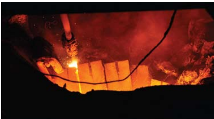
Cold face welding on a crown.
