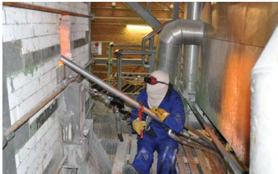
Welding being executed.
