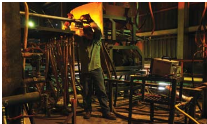
Welding via a monitor.
