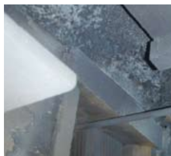
Transition brick port neck after ceramic welding.
