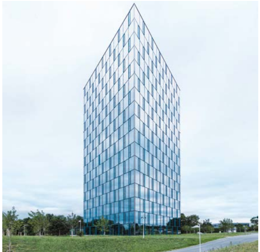
A flagship project: the building envelope of the new Festo Automation Center consists entirely of climate-active glass, adding a touch of modernity and prestige to this new building. Photo: Festo
