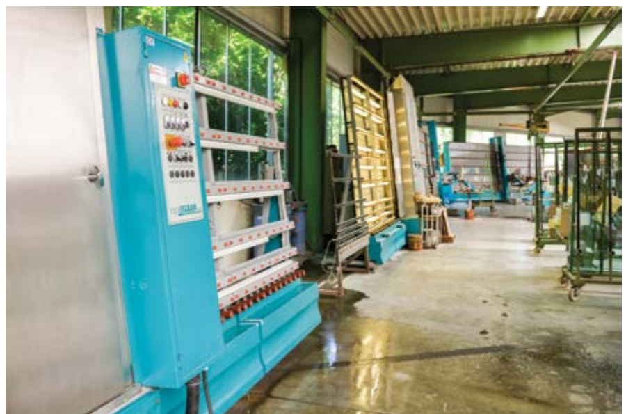
SCHRAML technology in glass processing: This innovative mechanical engineering company has been trusted by NOWAK for 15 years now. All the interfaces are from A+W.
