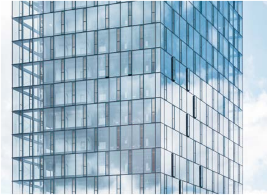
Energy efficiency: the glass façade of the new Festo Automation Center has been designed as an exhaust air façade. Using electrochromic window panes, it adjusts itself automatically to the prevailing lighting conditions. Photo: Festo
