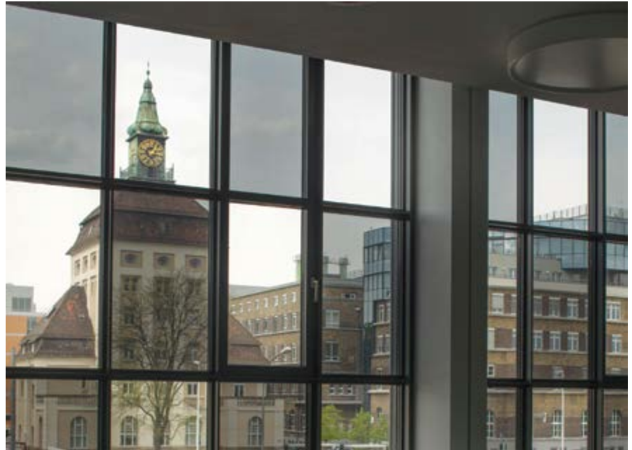
A coloured view: the windows at the Merck Innovation Center in Darmstadt contain liquid crystals which switch from light to dark and back again within seconds. Photo: Merck
