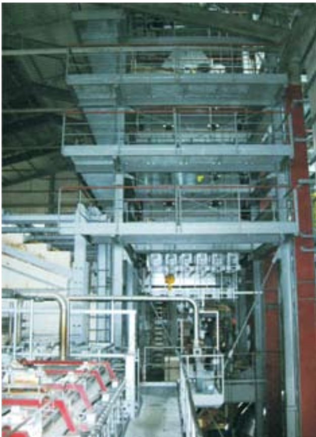
Figure 5 : Production Preheater 250t/d
