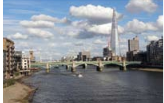
The Shard, the latest example of architectural glass innovation in London.
