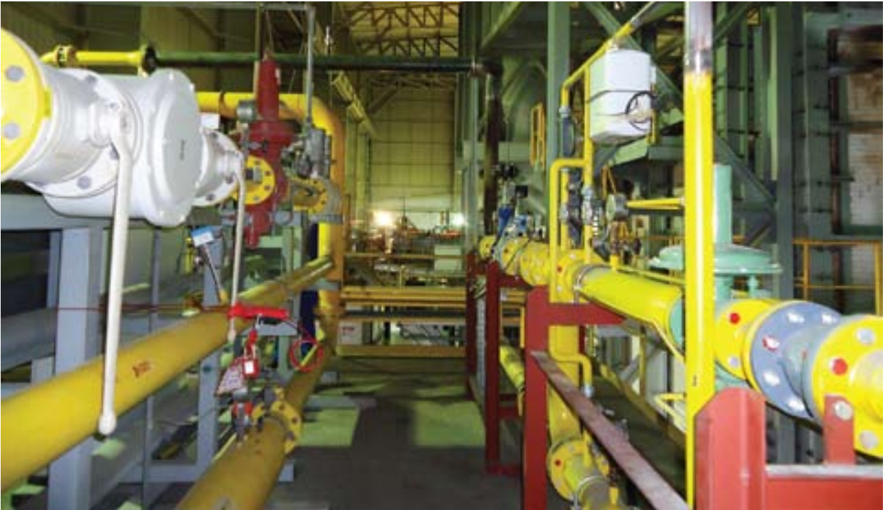
Gas stations for supplying biogas into a glass melting furnace.
