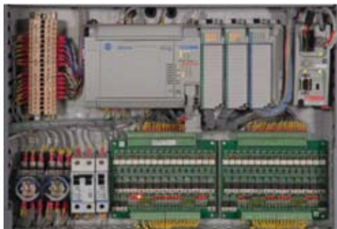
Assembled view of PLC unit, output cards with relays & MCB for Single Section of Timing System Panel
