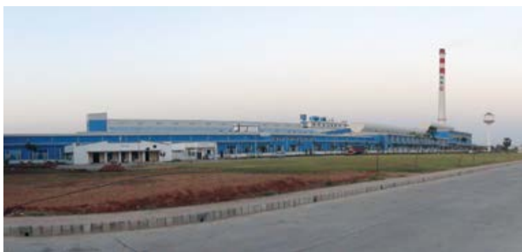
The HNG Float Glass Ltd plant occupies an area of 120 acres at Halol, Gujarat.
