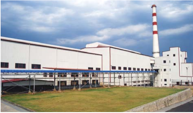
A dedicated 470 tonnes/day float glass production facility is operated at Roorkee, Uttarakhand.
